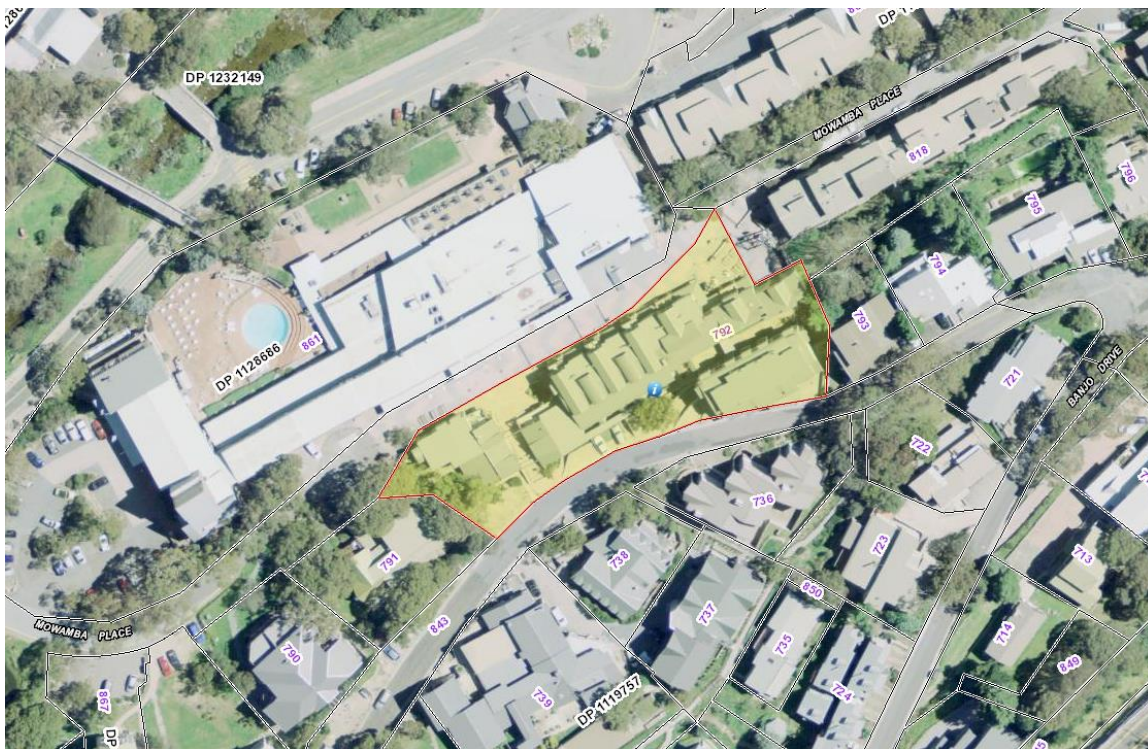
Figure 1: Aerial view of the subject building in context of the locality
